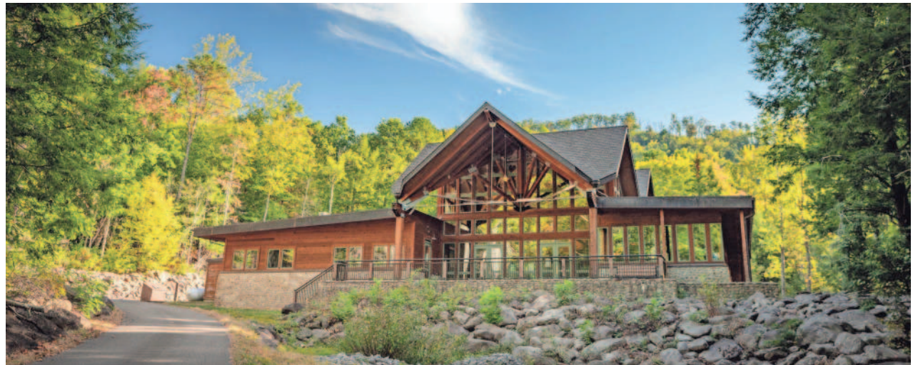
The facilities at Twin Creeks Science and Education Center in Tennessee include offices, a wet lab, natural history collections, and work spaces for visiting researchers. PROVIDED BY JOYE ARDYN DURHAM
